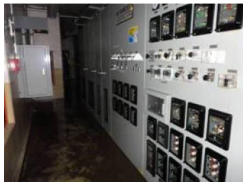
Fig. III-2-11(b) Damage of Fukushima Dai-ni NPS due to the tsunami.
