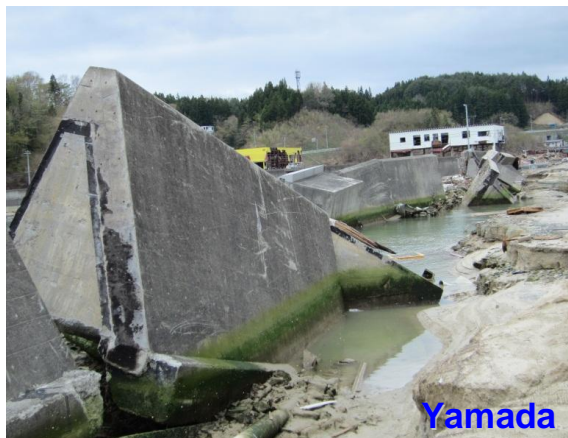
Destruction by tsunami scouring
