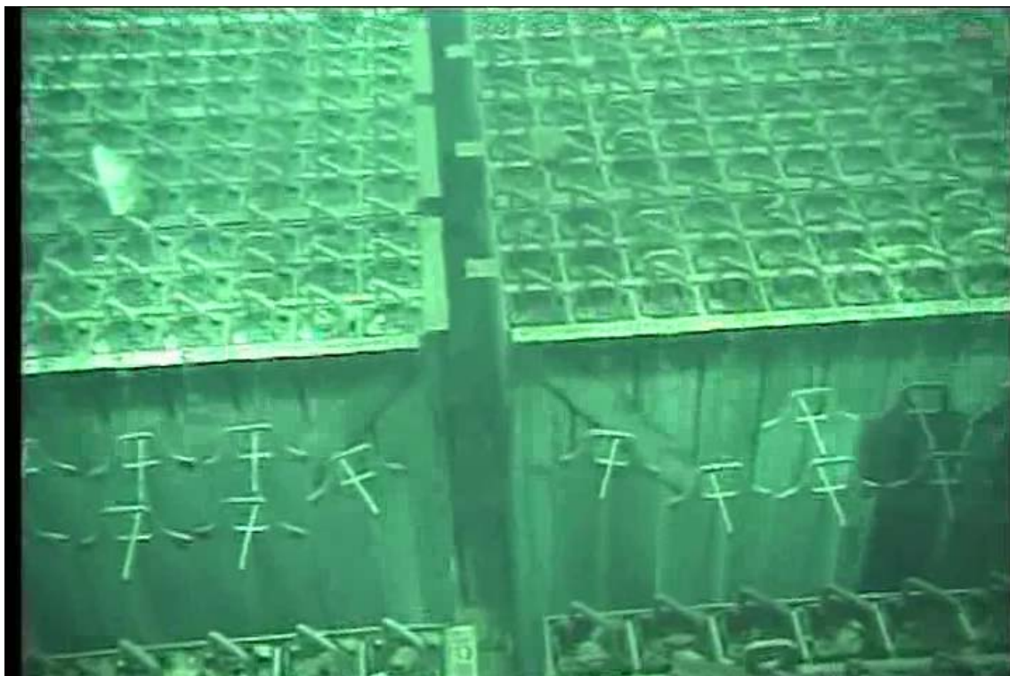
Figure II-2-48 Unit 4 Pool Viewed from Underwater (No. 3)
