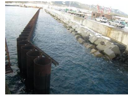
Photograph 4 Steel Pipe Sheet Pile (Example)
