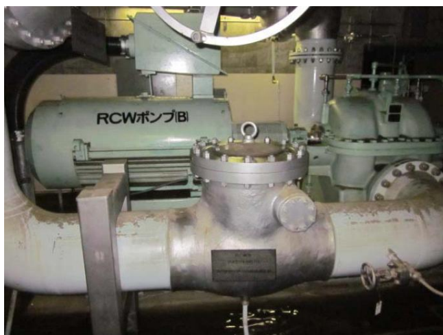
RCW pump (B) (after seawater was drained)
