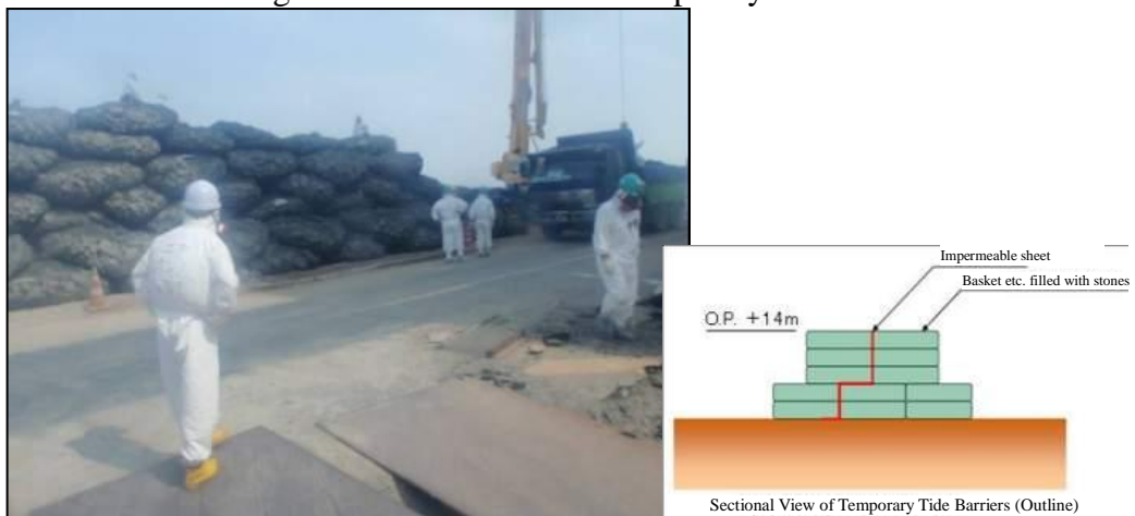
Fig. III-1-8 Installation of Temporary Tide Barriers
