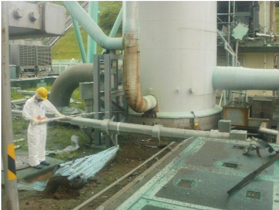
Location: Near the standby gas treatment system pipe joint at the bottom of the main exhaust stack of Units 1 and 2 Time: August 1, 2011, around 14:30 Photographed by: TEPCO
