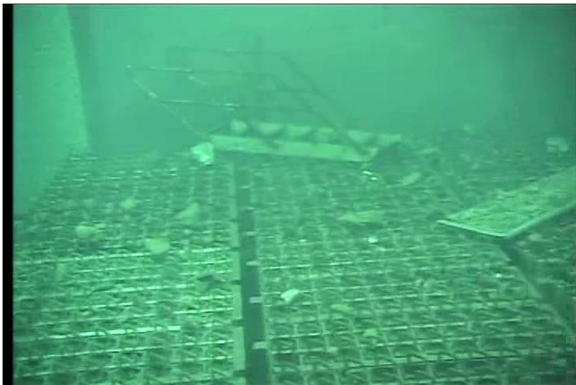
Figure II-2-47 Unit 4 Pool Viewed from Underwater (No. 2)
