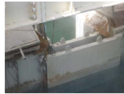
Spent fuel pool gate
